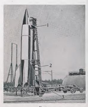
Fig. 49 1. Upper working platform 2. Lower working platform 3. Compressed air cylinder
