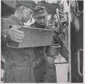
479. When the liquid reaches the mark on the measuring tank inspection window, showing that 126 litres have been tanked, the man at the measuring tank orders : HALT. The three-way cock on the measuring tank is closed.
